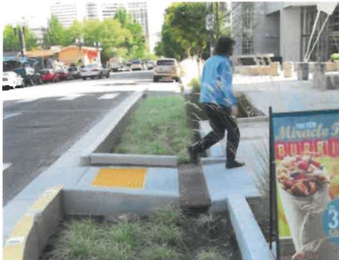
GSI curb extension
