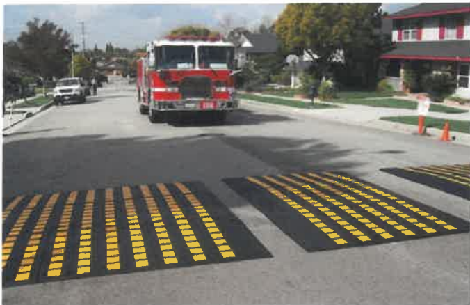
Example of an interim speed cushion
