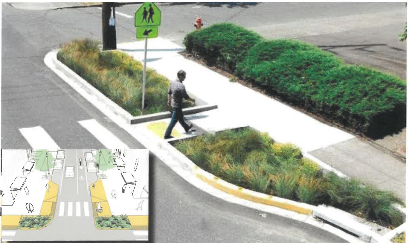
Figure 46 Curb extension with GSI
