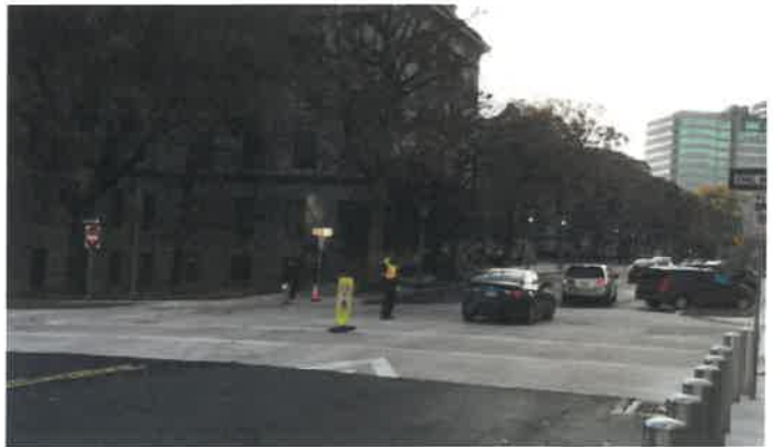
Raised intersection, Harrisburg, PA
