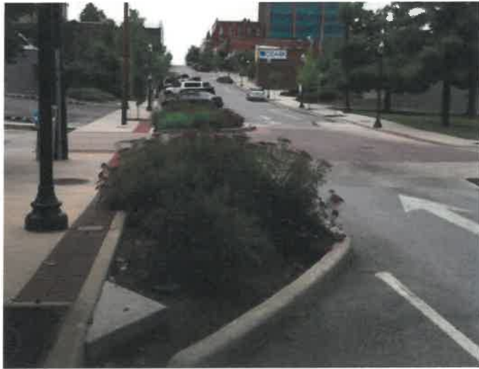
Green stormwater bumpout
