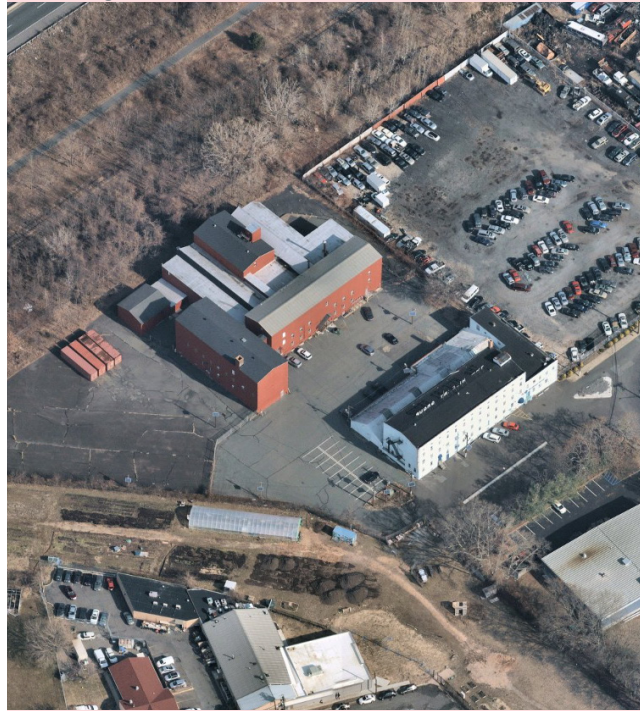
Coalport Works Buildings still exist
